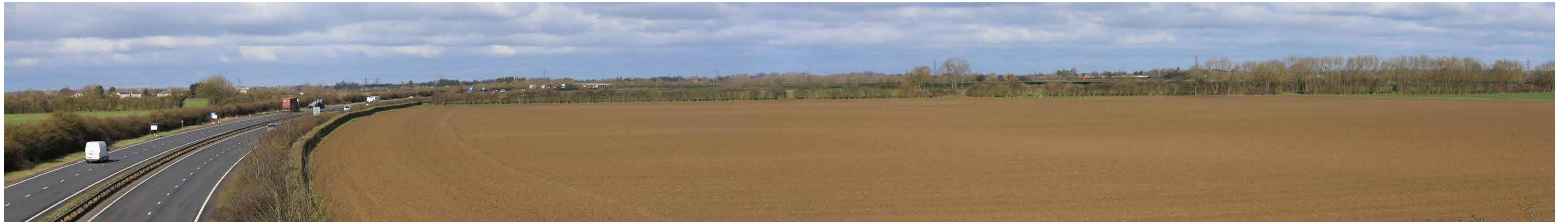
Current view from Low Fen Drove Way Bridge
