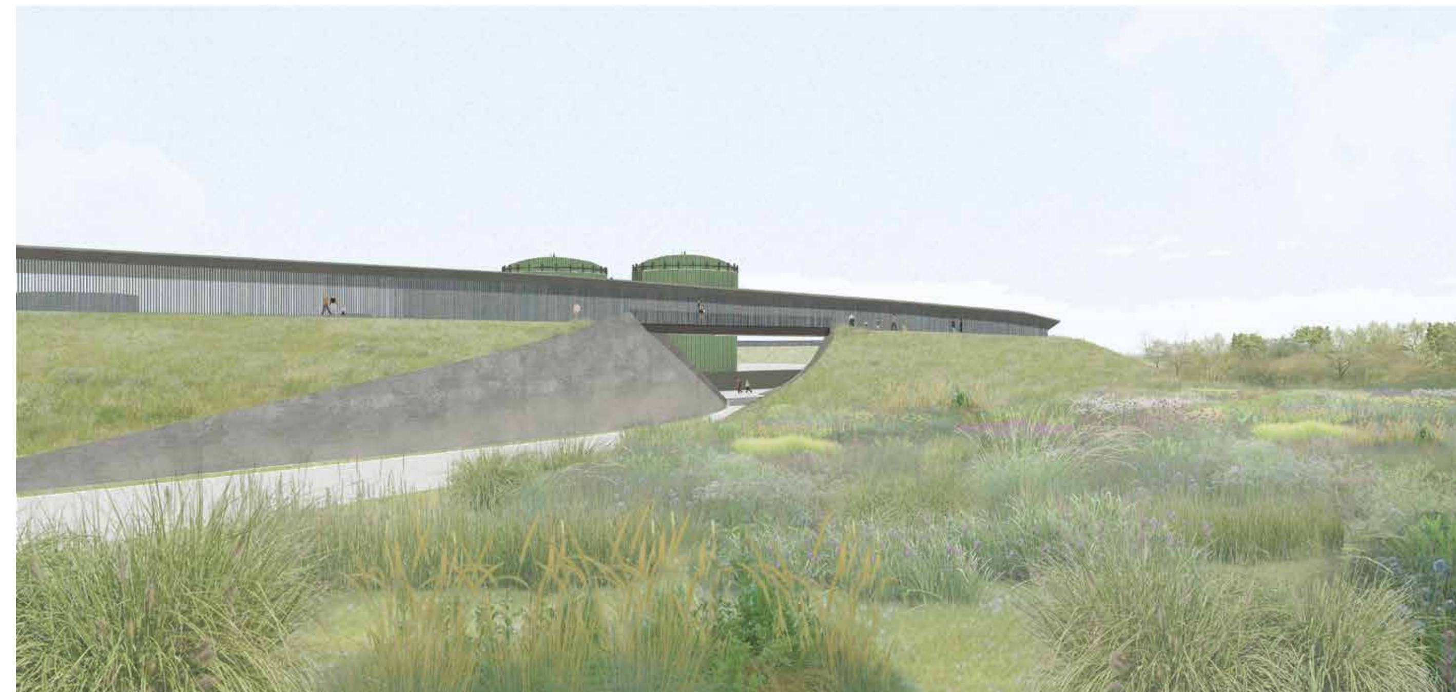
Illustrative visualisation of the anaerobic digester cladding with a natural, matt finish behind additional screening on top of the earthwork bank
